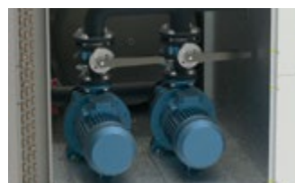
Pump section with or without storage tank.
